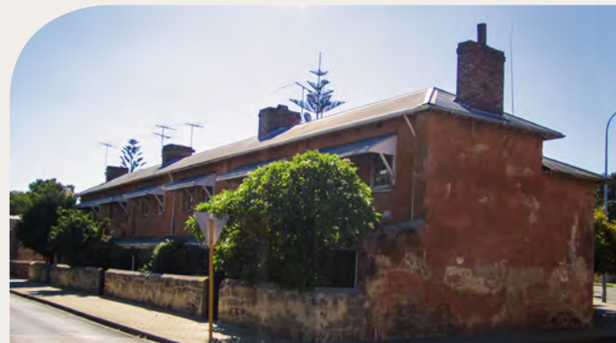
ABOVE: Warders' Cottages, Fremantle (1851-1858)
